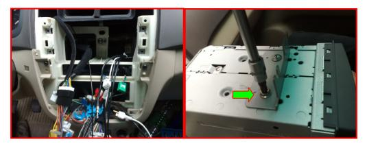
5. Connect the cables to the interface on the rear of the main unit ,then fix the main unit.
